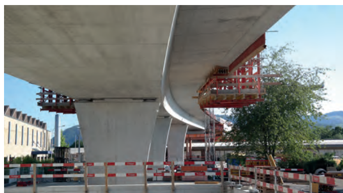
Neue Aarebrücke Bypass Thun Nord
